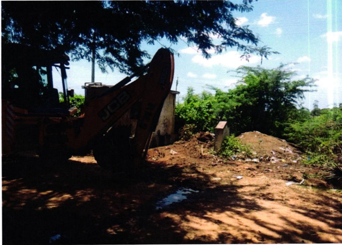
Clearing the waste at Dekkalivaripalem 2019
